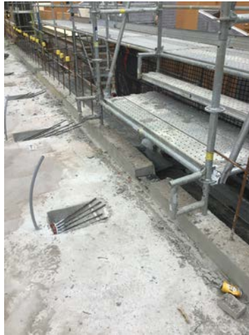
BLD A Level 4 - Additional step required
