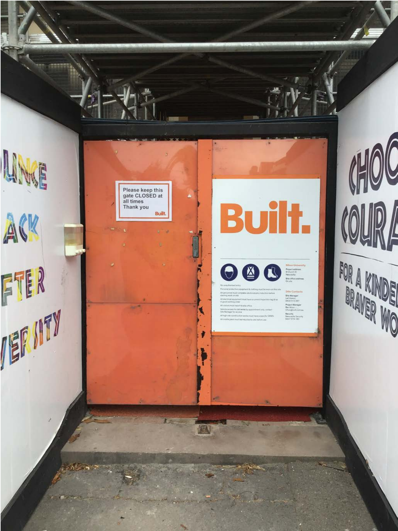
Site personnel gate with project signage & sanitiser station.
