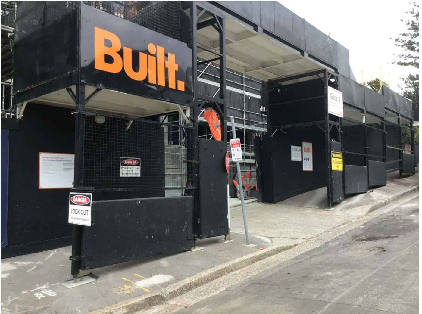
BLD A Gate with signage and no damage or graffiti
