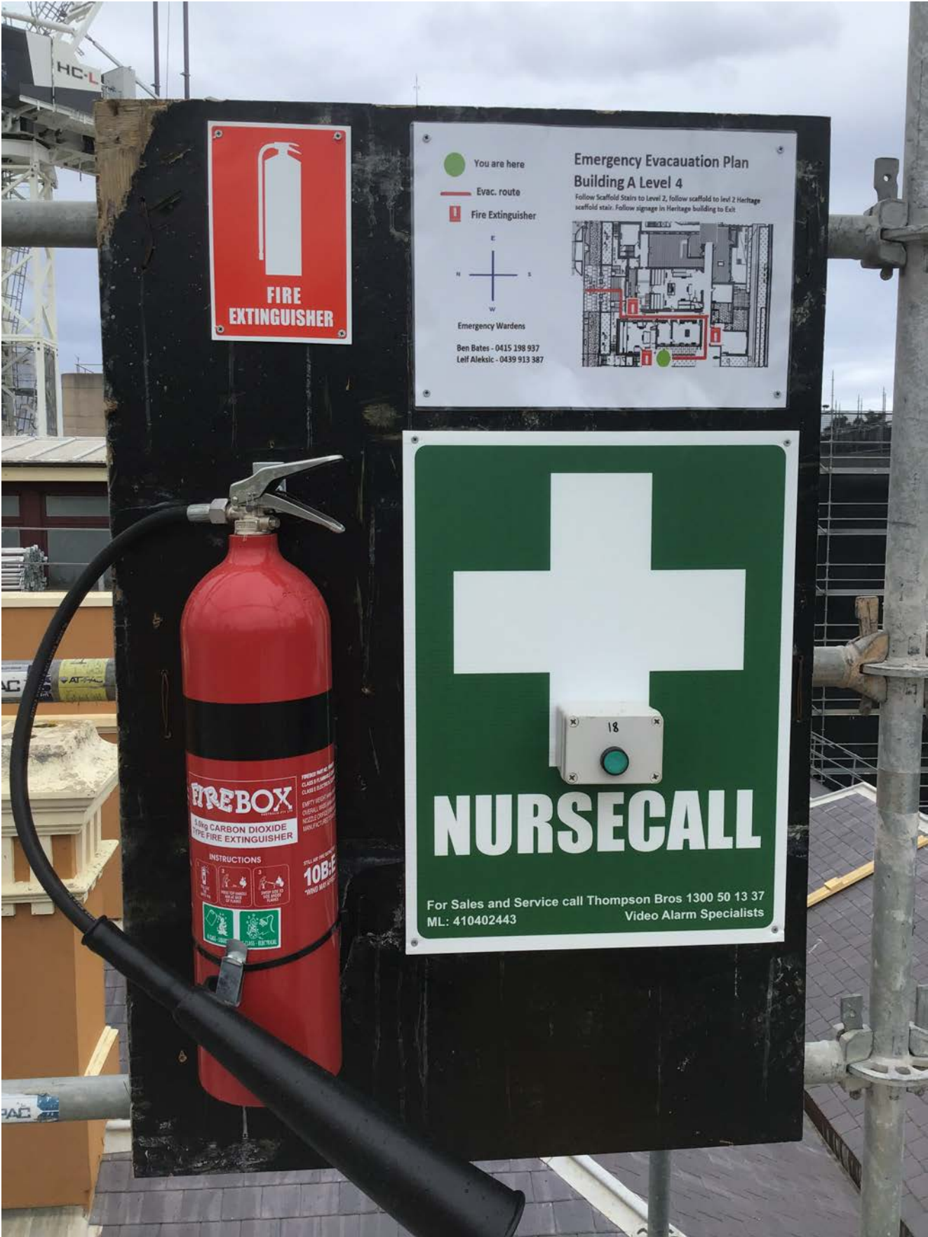
BLD A Scaffold - Safety Station on Level 4
