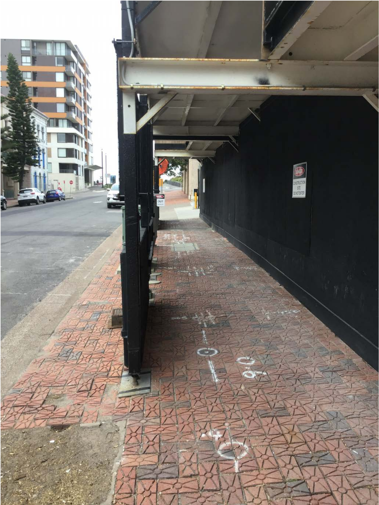
Church St footpath clean and clear. Hoarding in good condition.
