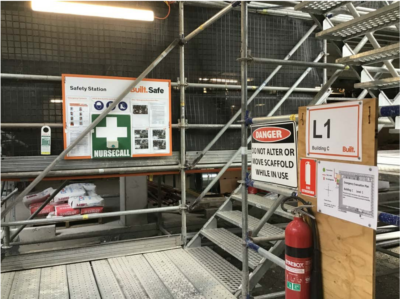
BLD C Scaffold - Safety Station & Signage
