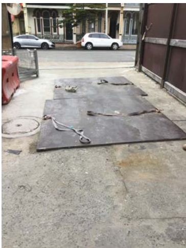
Road plates with slings attached stored in the driveway. Slings exposed to weather & traffic.
