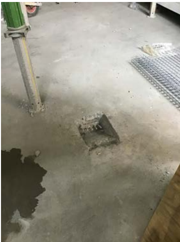
BLD B Level 2 - Pockets to be filled.
