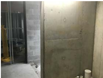
Stair C2 Level 4
