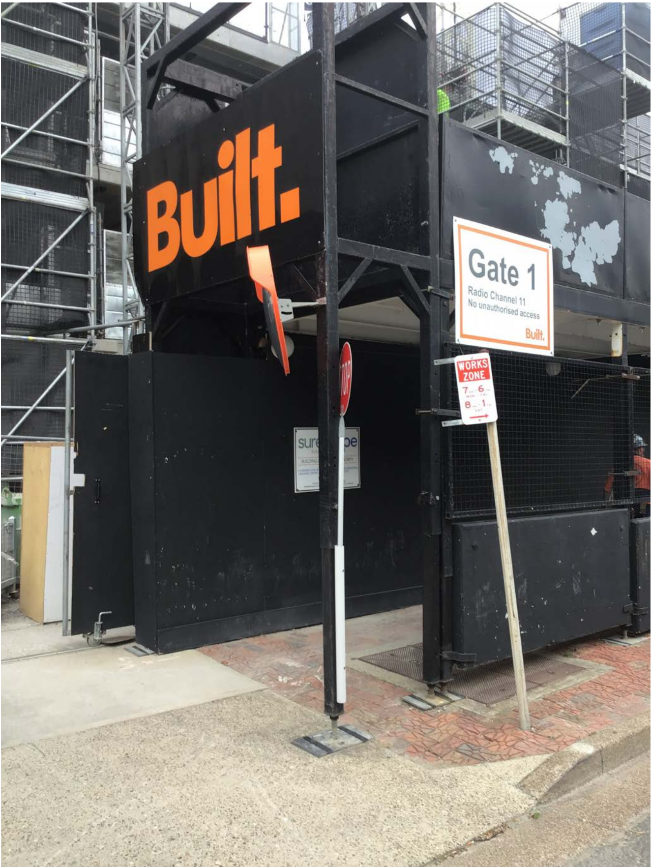
BLD C Gate with signage and no damage or graffiti
